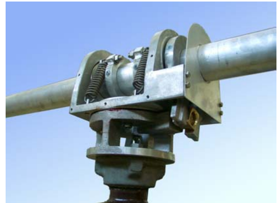
Double-break Disconnecter SDB rotating mechanism of current path
